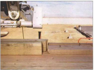
rafters. A beam saw is just an oversized circular saw; my Makita has a 16in. blade. So if I'm cutting blocks from 2x4 or 2x6 stock on edge, the entire cut can be made in a single pass. In this case, I place a flat 2x under the stock near the chalkline to hold the 2x material away from the deck (top photo, facing page). A little paraffin on the blade makes the cut go easier.
